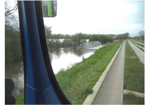
The whole alignment of the Greenway between Swavesey and St Ives is prone to flooding, but the busway itself is generally expected to not flood.
